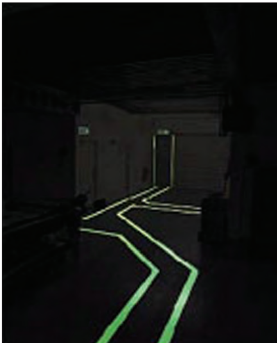
Figure 56: A way-guidance system
